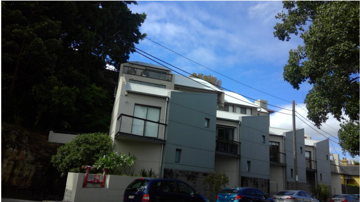
Figure 1: View of development known as 66-82 Palmer Street looking from northern end of the building.
